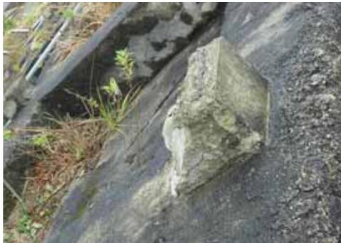
(a) Ground anchor head broke
