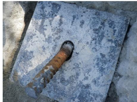
(b) Rust on the ground anchor (rod type)
